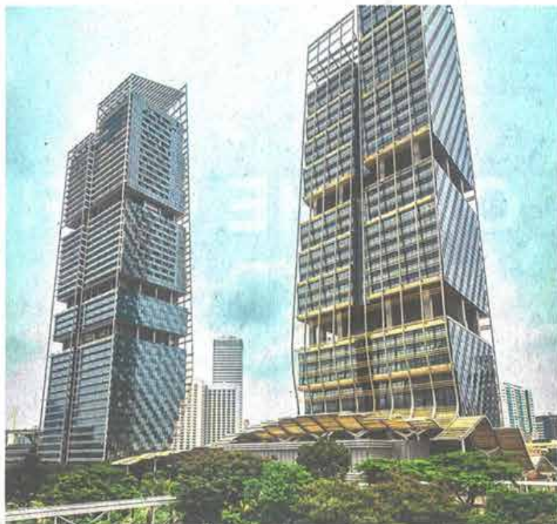
South Beach has a sustainable microclimatic canopy which covers the open spaces within the development.
